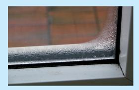
The water **must be wiped away**, so that this moisture does not need to be ventilated via the room air.
